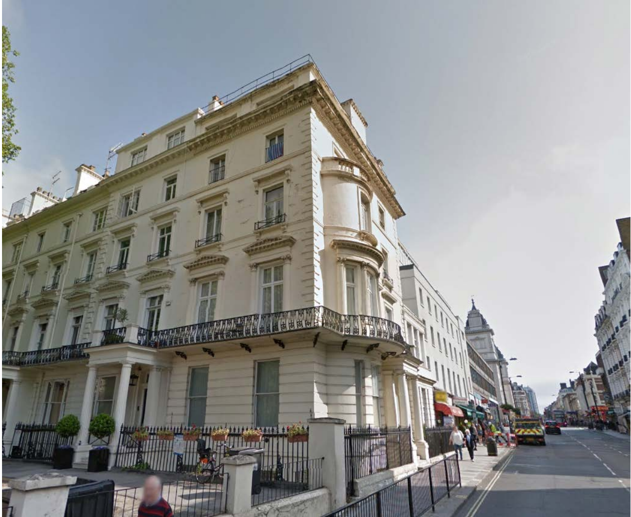
View of building from Westbourne Terrace.
