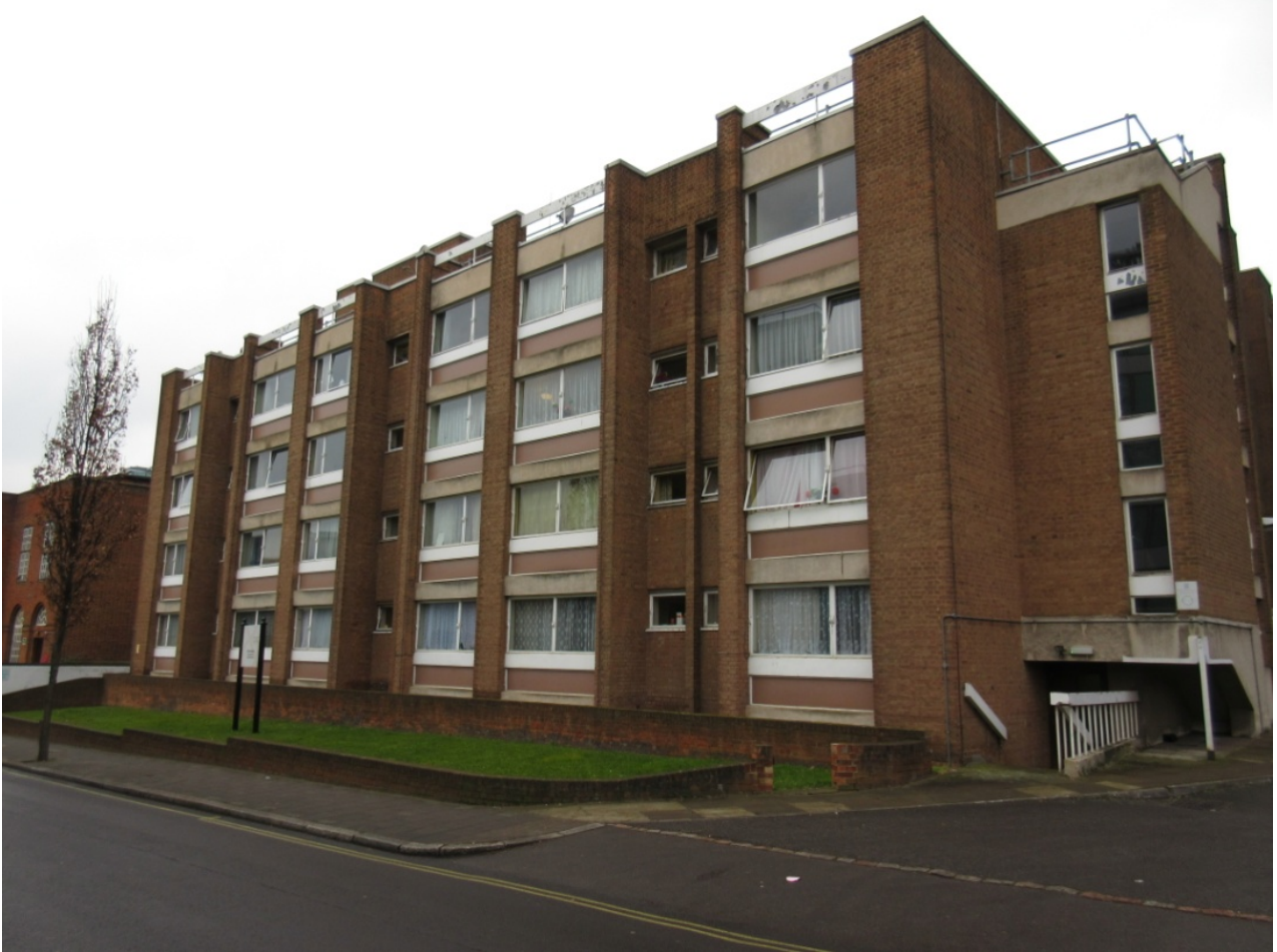
EXISTING LODGE ROAD ELEVATION
