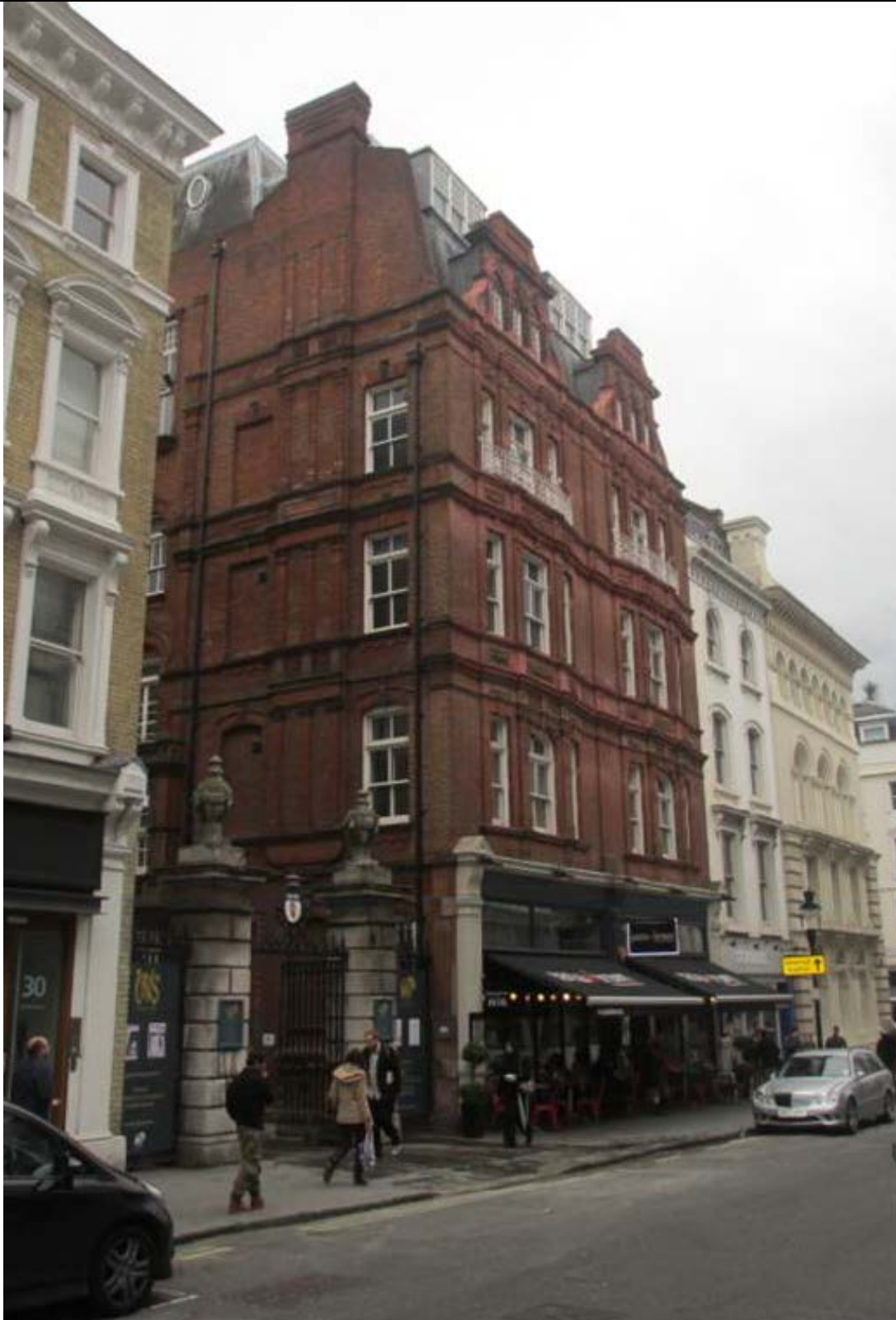
View from Bedford Street
